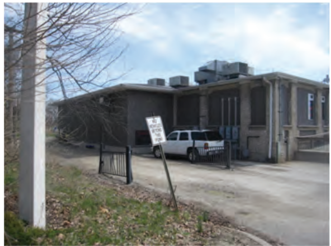
Beach House Rear
